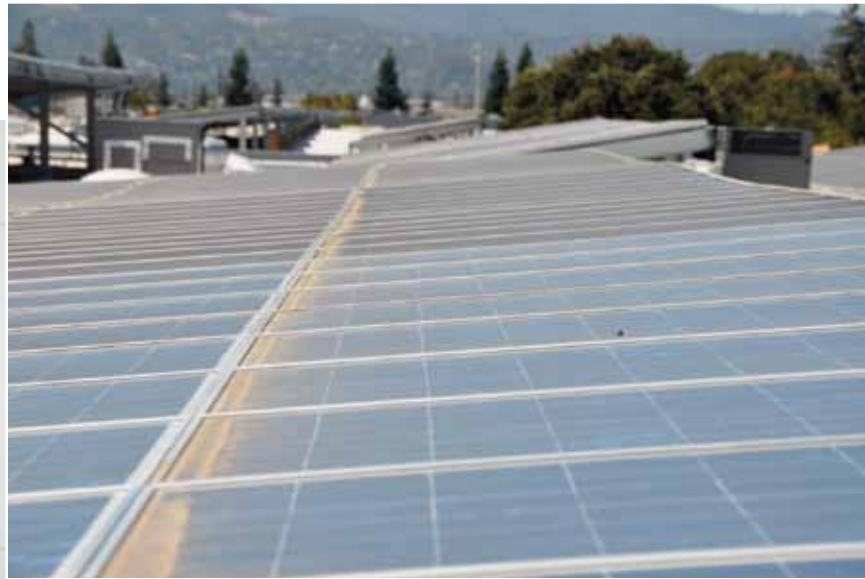
PURETi's photocatalytic solutions keep building surfaces (left, with the treated segment on the left), solar panels (above, with treated cells in the foreground), and windows (right, with treated windows toward the middle) free of grime—reducing maintenance costs, increasing efficiency, and providing all of these surfaces with air purifying capabilities.
