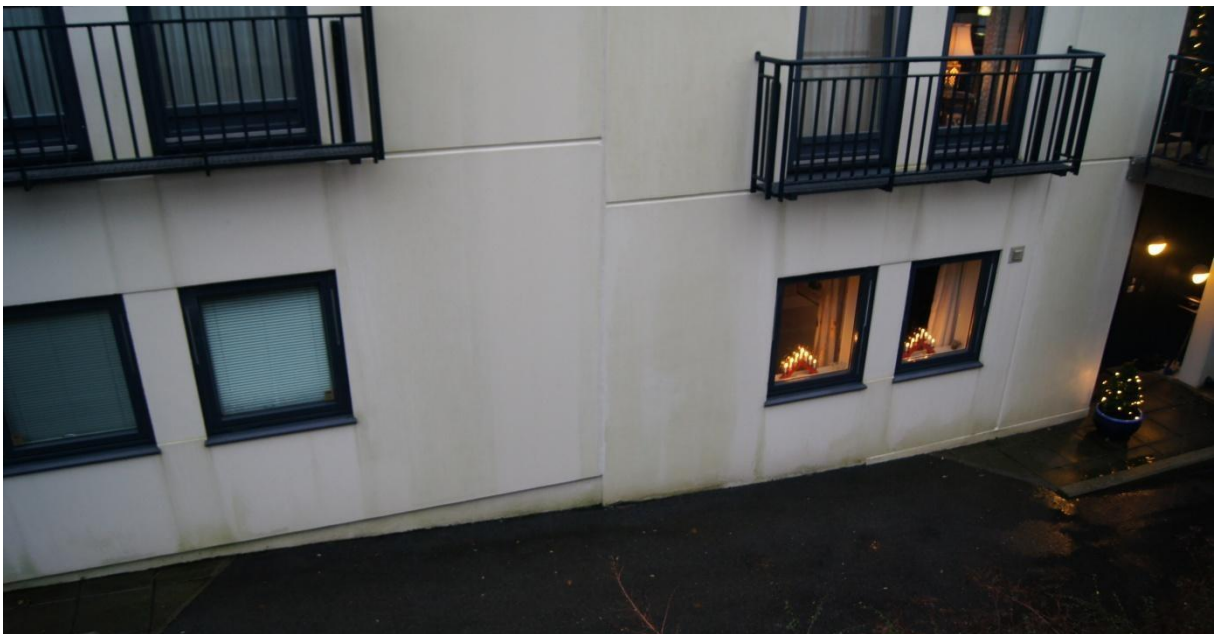
Test area after 6 months. The test area is still clean and nice, while the surrounding area has a clearer green color from greenery and acid rain.
