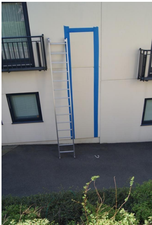
Test area masked, washed and ready for application.
